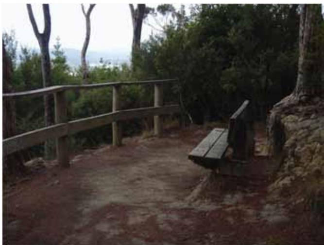
Before the upgrade (Photo taken on Feb 2010)
